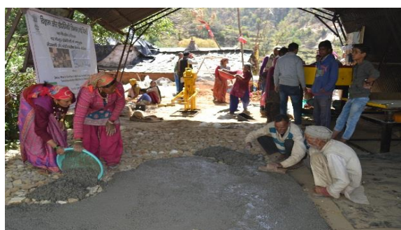
Floor preparation and levelling of land for stacking of freshly de-moulded SCEB
