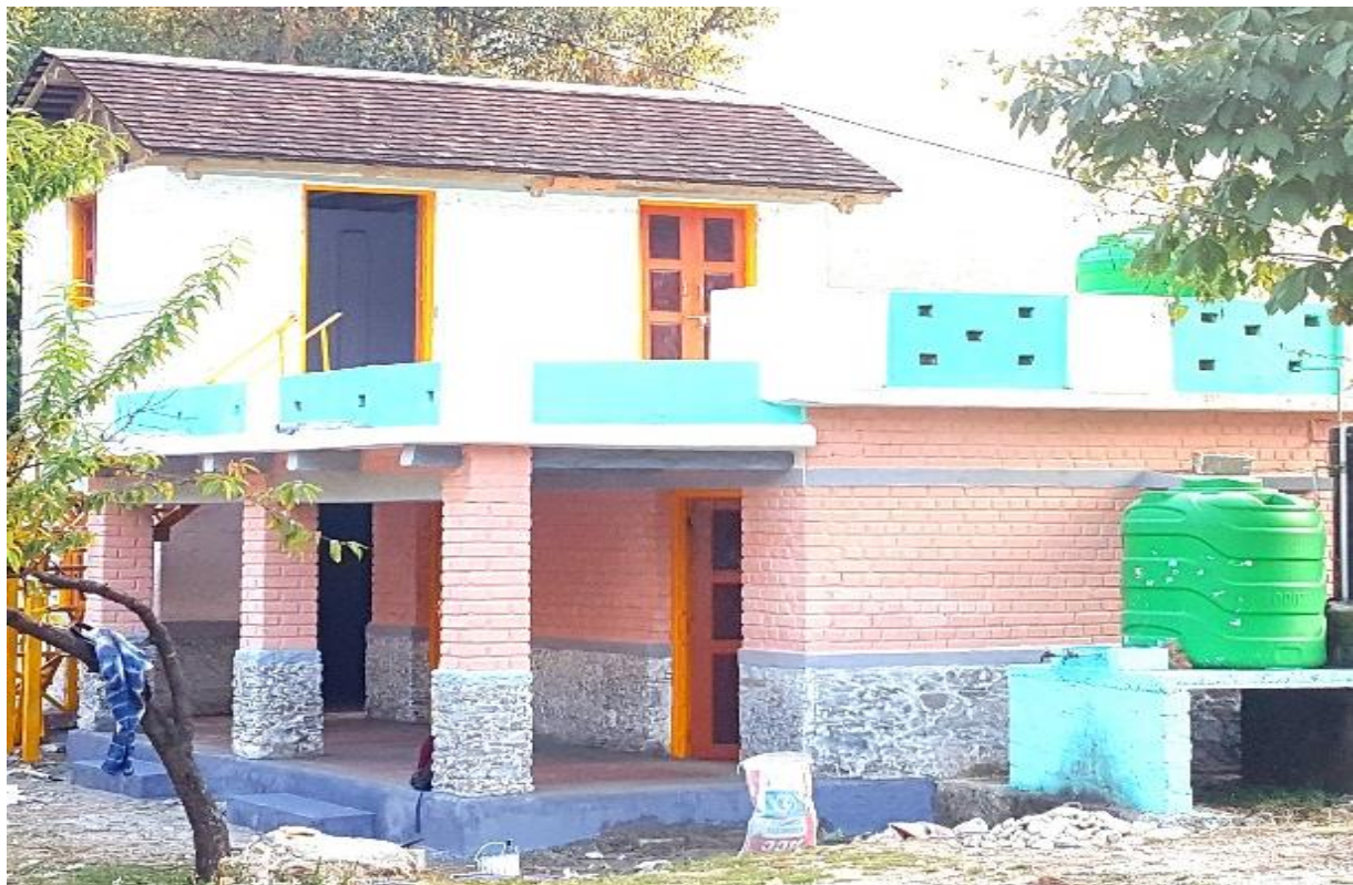
SCEB wall finish in lime plaster and paint in Community building, Kamad village, Uttarkashi
