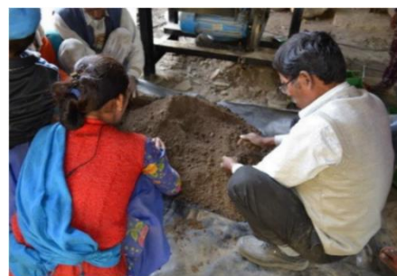
Preparation of SCEB mix by hand
