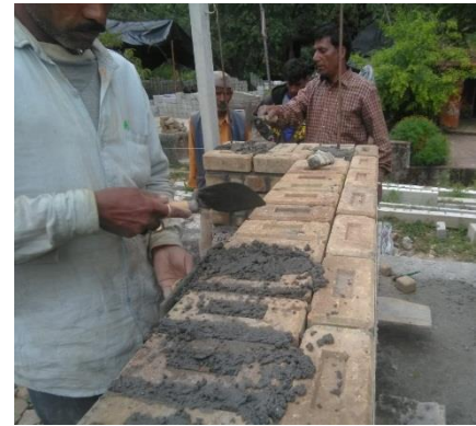
Masonry in English bond
