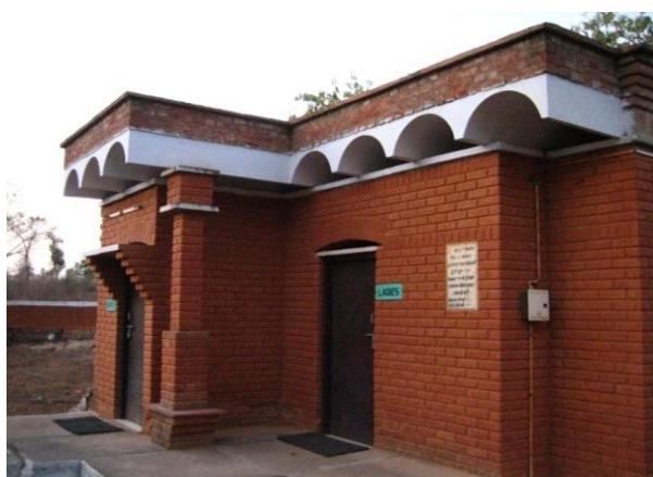
Building using SCEB at TARAGram Madhya Pradesh
