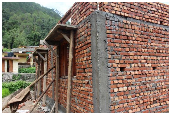
Red burnt clay bricks masonry in houses of Kamad village, Uttarkashi
