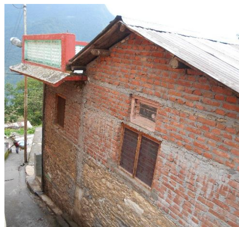
Use of red burnt clay bricks in combination with stone masonry in one of the houses in Raithal village, Uttarkashi
