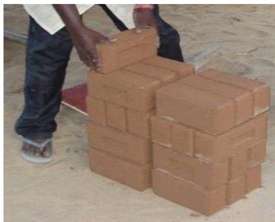
Step-8: Transfer the blocks at the stacking yard for curing.
