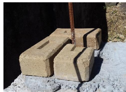
Brick placement around RCC infill
