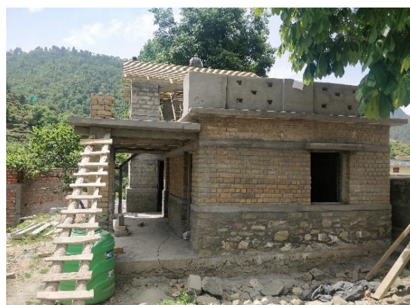
Community building in Kamad village, Dunda block in Uttarkashi
