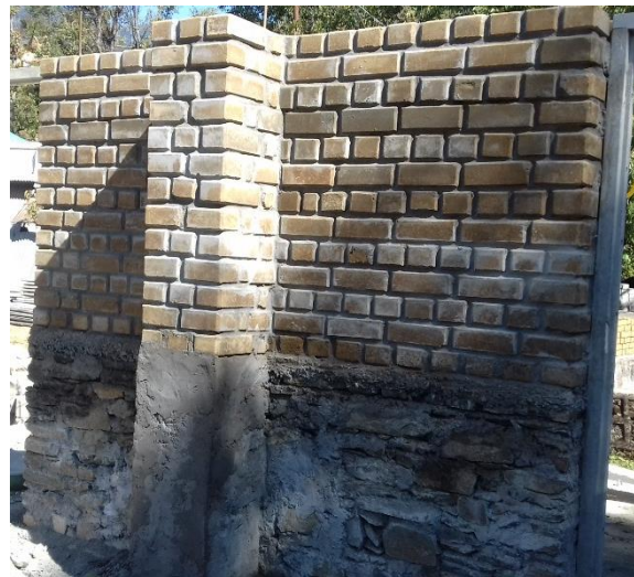
SCEB Masonry over Random rubble masonry in Community building at Kamad village, Uttarkashi.
